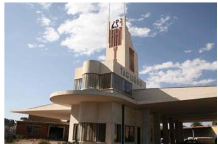
The Fiat Tagliero building in Asmara
