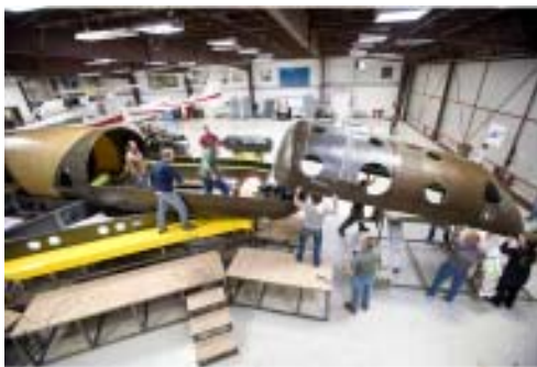
WK2 under construction
