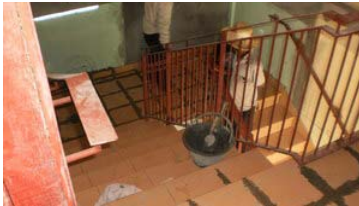
2nd floor view of the new stairs
