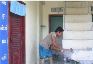
Tearing down the old stairs
