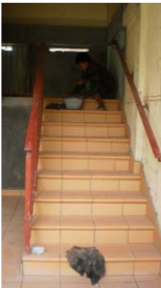
The new stairs
